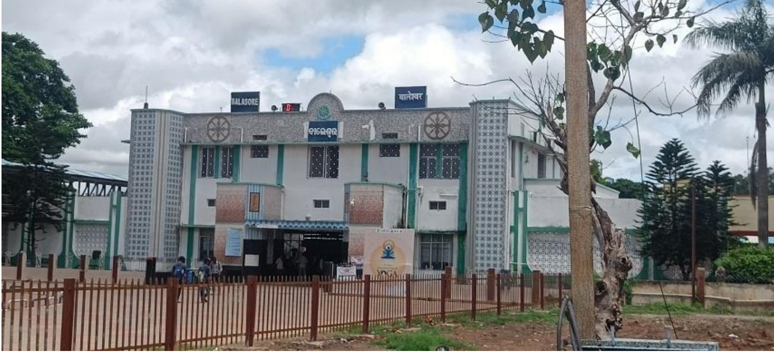
1. Main Station building
