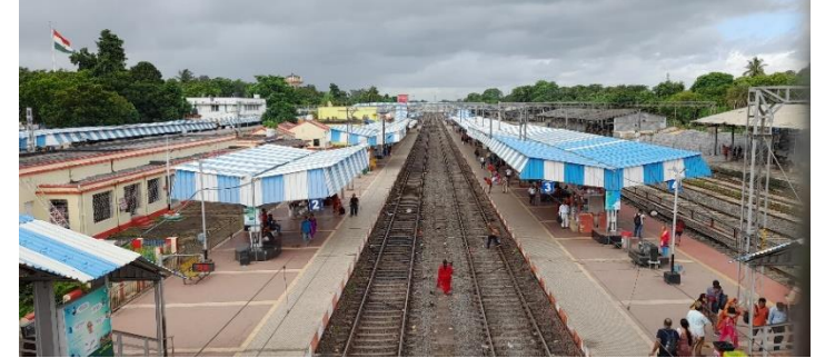
2. FOB towards Howrah side
